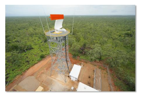
Working in close association with the design & construct team, **idetail3D** were required to be flexible with design changes and attentive to transport and buildability issues. Due to the remote location, many intricate components were included as part of the structural steel model to address problems in-office before they eventuated on site.
