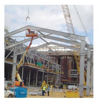
To accomplish minimal welding in the structure, clip angle connections were used instead of end plates on beams. In place of welding bracing cleats to beams and columns, they were fabricated separately and bolted in place. This allowed almost the entire structure to be fabricated using beam line machinery, eliminating many man hours of welding, as well as possible human error in fabrication.
